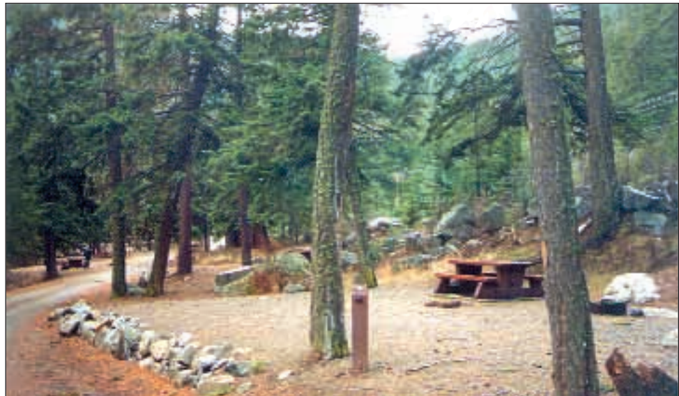
Vaseux Lake Provincial Park (left). Sites can direct construction through what they provide. This example shows a split level campsite: the vehicle high, the picnic table and fire iron lower, and at natural grade the beach. The rocks retaining the parking spot simply join two existing rock outcrops. In the background, the rocks set in a curve that retains the campsite can just be seen. Native vegetation frames the views and creates the spaces.
