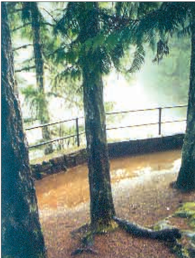
Englishman River Falls Provincial Park (below and right). Viewing the waterfalls from this terrace, rather than a platform, allows simpler, less obtrusive construction and reduces maintenance. The stone plinth and black metal rails create a permanent appearing facility, which has become part of the park rather than an addition.
