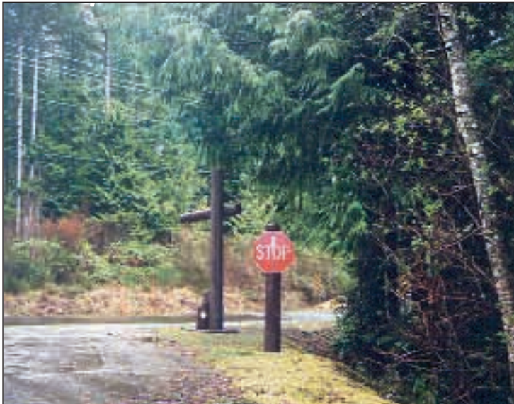
China Beach Provincial Park (left). This BC Parks entry sign and traffic sign both have landscape scale wood posts with the same finish. All information is important for visitors, and this is a simple way to achieve a unified style for signage.
