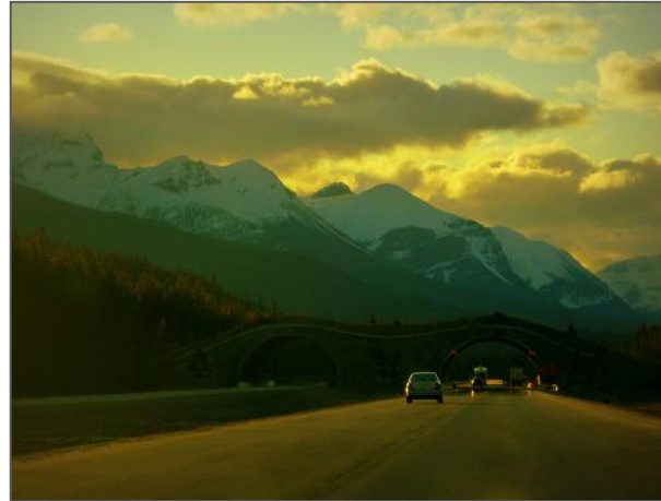
Wildlife overpass, Trans-Canada Hwy, Banff, AB. Credit: Anita Sott, 2012.
