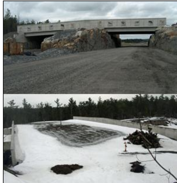
Image 1.4: Hwy 69 wildlife overpass as viewed from road with images of deer and moose sculpted into side (top); overpass surface landscaping in progress (bottom). Credit: Kari Gunson. Source: CBC News, 2012.
