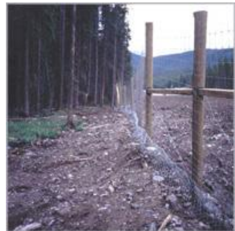
Image 5.3: 2.4 m high fence with buried apron. Credit: Tony Clevenger. Source: Parks Canada, 2011.
