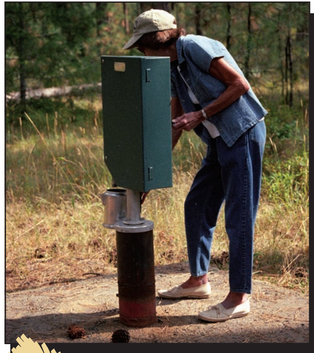
Figure 71—This accessible handpump is operated by a crank, making it possible for almost everyone to draw water independently.
